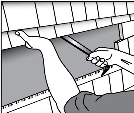
Pry the nails out of the nail hem of the damaged panel.
