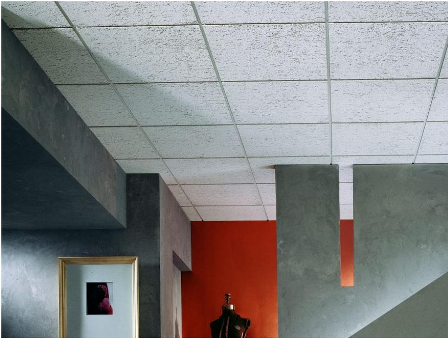
A perfect choice for noisy environments, these durable, panels possess excellent sound control and noise reduction qualities. Glacier™ Basic, Frost™ Basic and "F" Fissured™ Basic Acoustical Ceiling Panels combine a high noise reduction coefficient and ceiling attenuation class that make them an ideal choice for environments where noise reduction is important. Perfect for conference and lobby areas, executive offices, hospitality environments, retail stores and transportation terminals.
