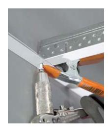
Armstrong Ceilings Wall Molding Connection (GCWA Clip – Non-Seismic)
