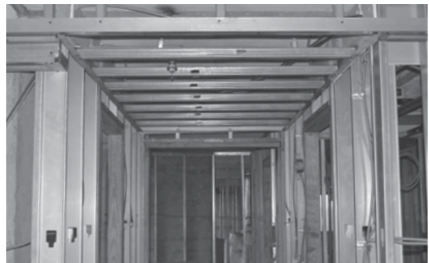
Corridor framing using traditional steel studs
