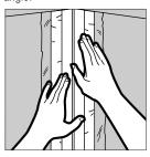
Use the knife (or a damp sponge) to remove excess compound, eliminating any air bubbles under the paper. Allow to dry.
