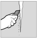
b. Apply compound to crack with 5" finishing knife.
