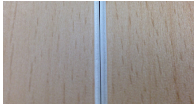
The depth of the groove should be two-thirds the thickness of the wear layer. Do not groove through the backing.
