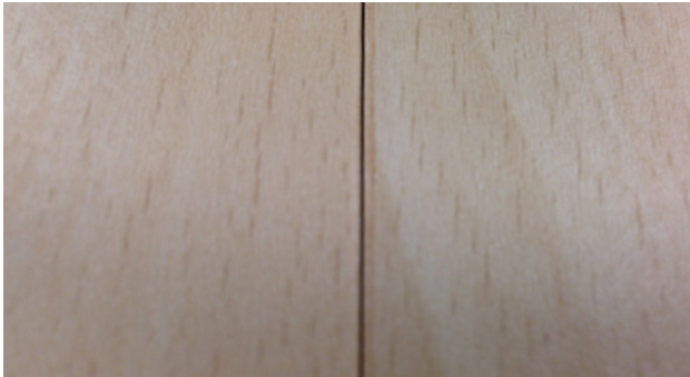
The seam should be cut with a maximum 1/64" gap. Approximately the thickness of a business card.
