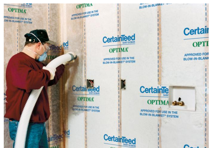
Figure 2. Installation of blowing wool in closed cavity application.
