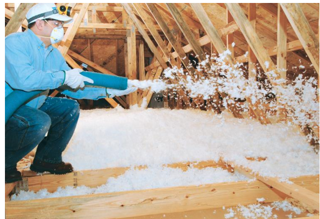
Figure 1- Installation of blowing wool in open cavity application.
