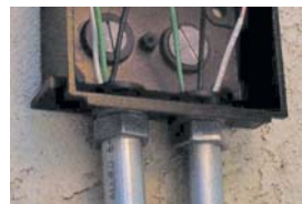
The WS option allows for mounting sconces using surface conduit. The sconce mounts over a factory supplied surface junction box allowing for use in retrofit situations or where surface conduit is required.
