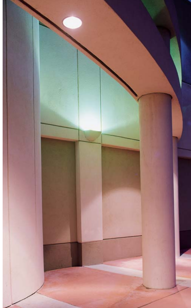
Tucking a sconce into discrete locations adds a dramatic effect, improving security and making the building come alive at night.
