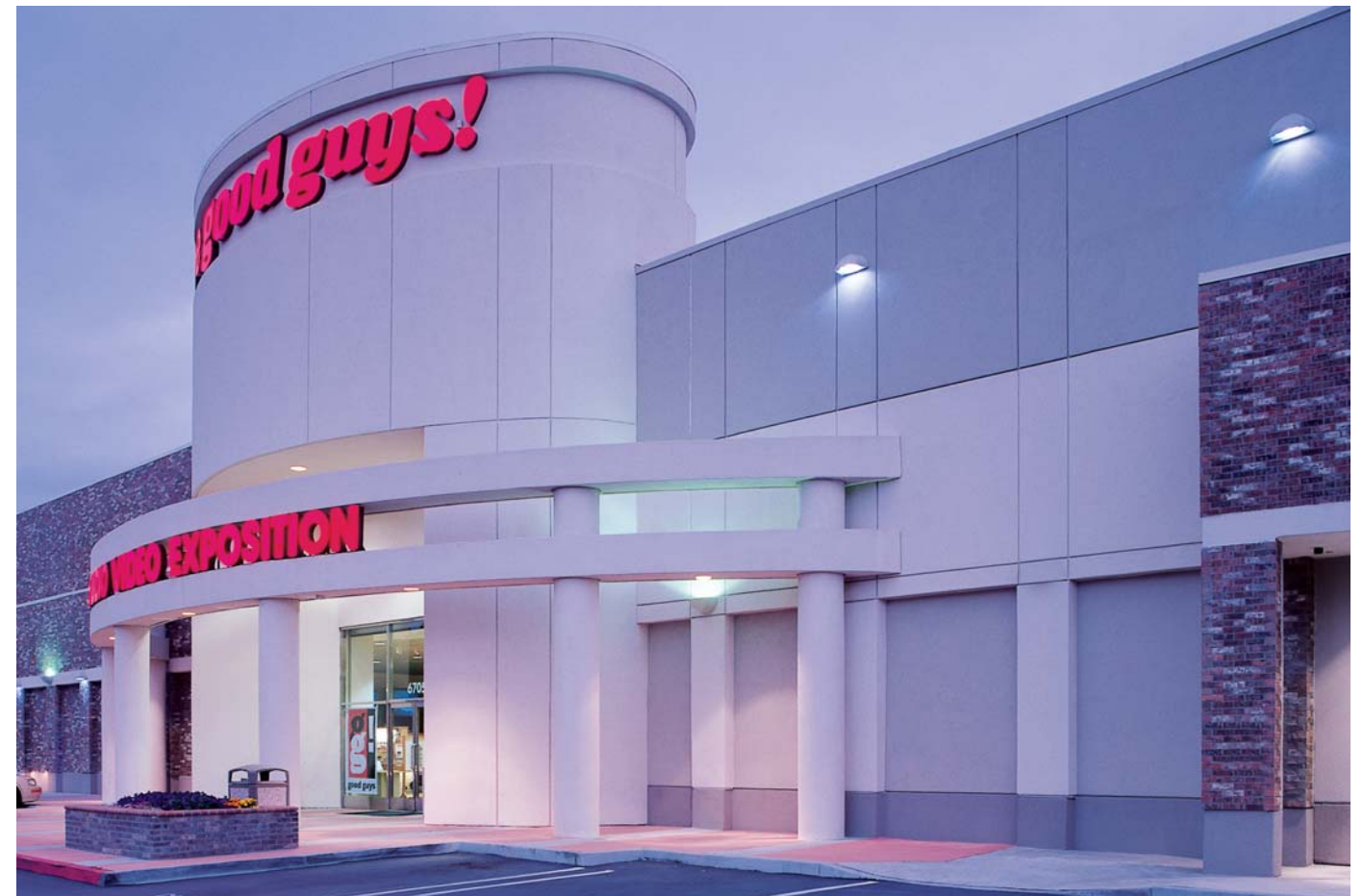
Combining standard downlight sconces with inverted sconces allows for the right amount of light in all the right places around the building.
