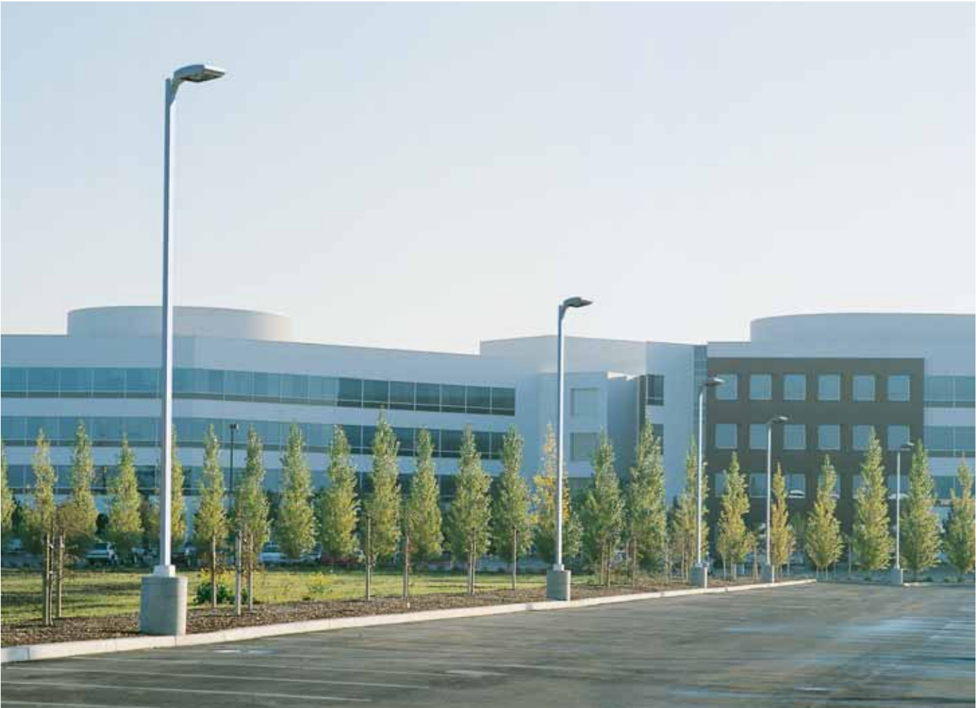
Of particular interest is the extended forward throw of the 4XL optical system, which enables exceptionally wide illumination patterns. Even at a mounting height of 24', Gullwing eliminates the need for cobra heads and unsightly mast arm extensions.
