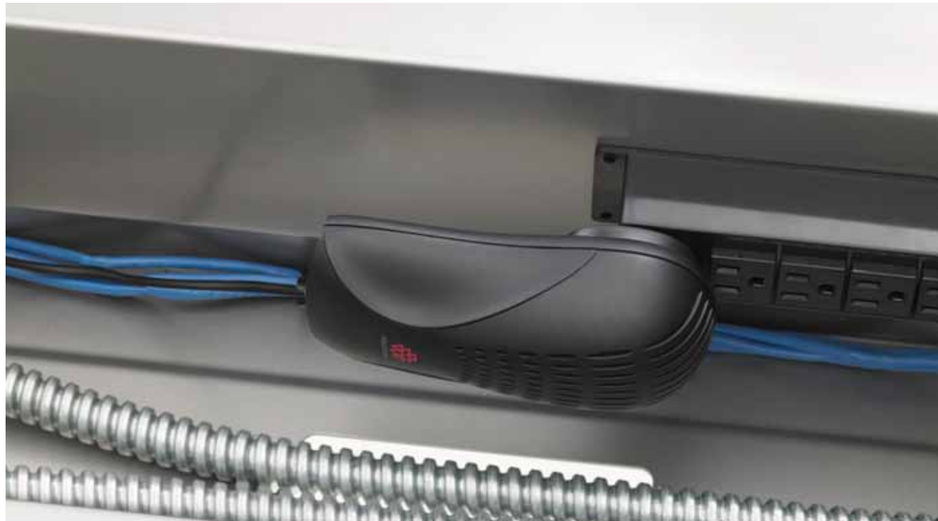
Auxiliary power strip inside power channel with Polycom™ power and network module connections
