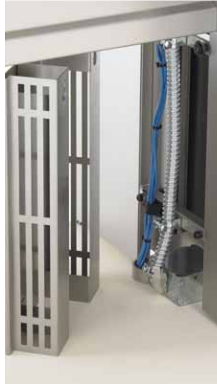
Core drill with floor mounted junction box
