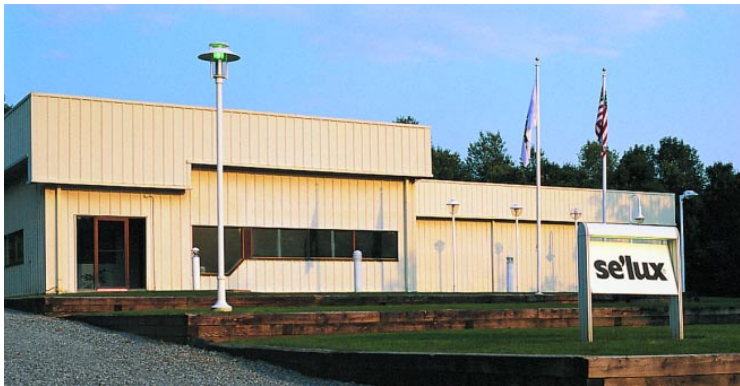
The SELUX full service manufacturing facility in New York.
