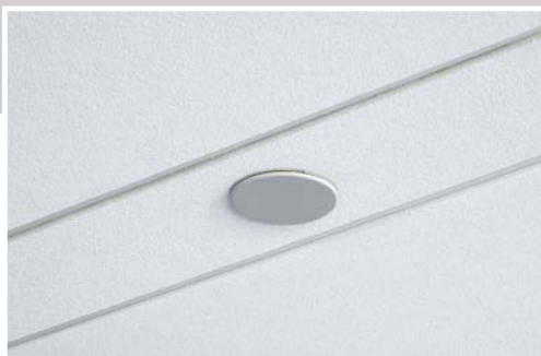
TechZone-compatible Sprinkler Systems
