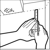
**Choose a ceiling height.** Allow clearance of at least 4" below the lowest air duct, pipe or beam. Snap a chalk line 3/4" above the desired ceiling height.
