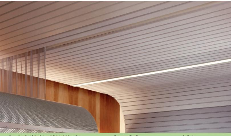
Paraline Linear Metal Ceiling System with Field-Applied Custom Paint
