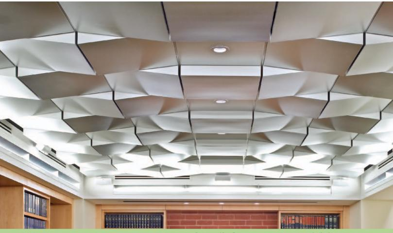
GEOMETRIX 3" Flat Panels and 3" Wedge Panels/ DONN CENTRICITEE DXT Suspension System
