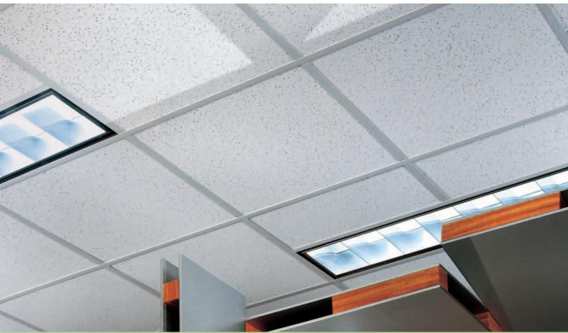
RADAR High-NRC Panels with *CLIMAPLUS* Superior Performance/DONN DX/DXL Suspension System
