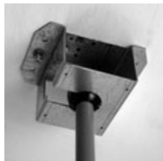
Hang straight bracket and pendant Figure B
