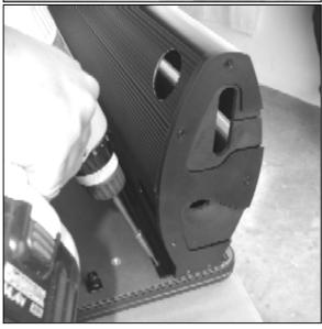
Install screws on both sides in every pilot hole
