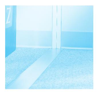
The 400 Series architectural joint systems are designed with centering bars that maintain plate position while accommodating seismic movement.
