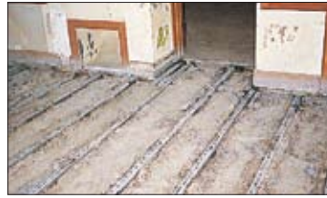
School classroom floor renovation using Dura-Cap. Close-up of wood sleepers, dips and pot holes before (above), and the new, smooth Dura-Cap floor after (below).
