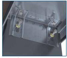
Attach SL to wall stud with provided screws through Step Bushings.
