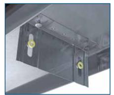
Fasten SL to top track at designed stud spacing with engineered fastener.
