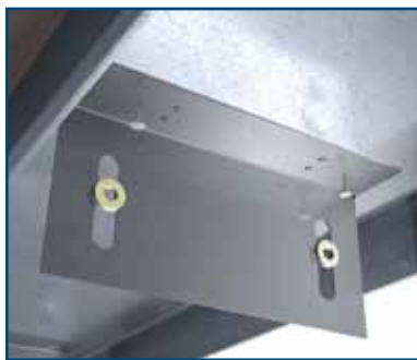
Attach VertiTrack VTD to deck with approved fasteners.
