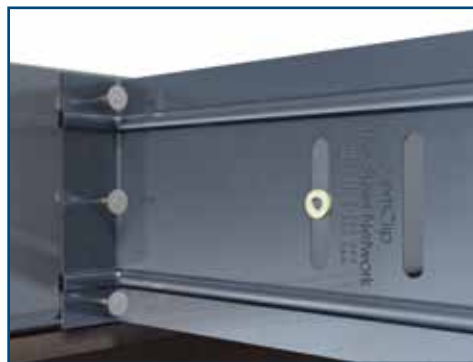
Attach SLB to structure with required fasteners.
