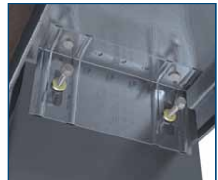
Attach SL to wall stud with provided screws through Step Bushings.
