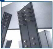
Attach StiffClip WC to framing member with required screws through guide holes.
