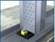
Place StiffClip TD at bottom of stud and attach clip to deck with approved anchor.
