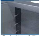
Place floor joist over StiffClip JC. Attach joist to clip with approved number of screws.
