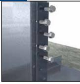
Attach StiffClip FS to wall studs with approved screws through guide holes.
