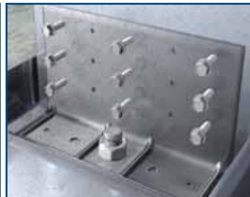
Secure clip to stud with required amount of symmetrically placed #12 screw fasteners.
