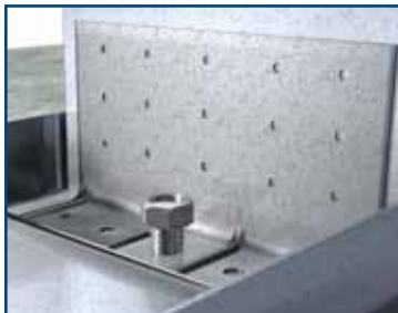
Attach clip to deck with approved anchor.
