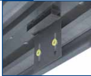
Twist clip into place within DriftTrak. Ensure stiffener is in place prior to installation.
