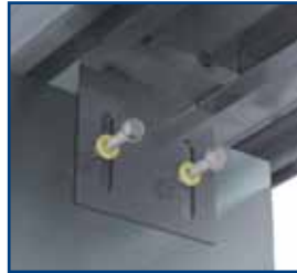
Fasten to stud using provided screws through Step Bushings.
