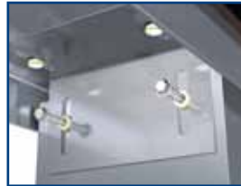
Attach DriftClip DSL to stud with provided #12 screws through each Step Bushing.
