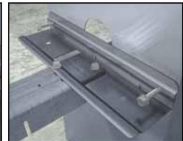
Secure clip to stud web and channel with #10 screws through guide holes (2 into web, 2 into channel).
