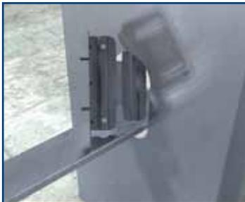
Twist BridgeClip into stud punchout and snap on BridgeBar or cold-rolled channel (CRC) with bottom tabs.
