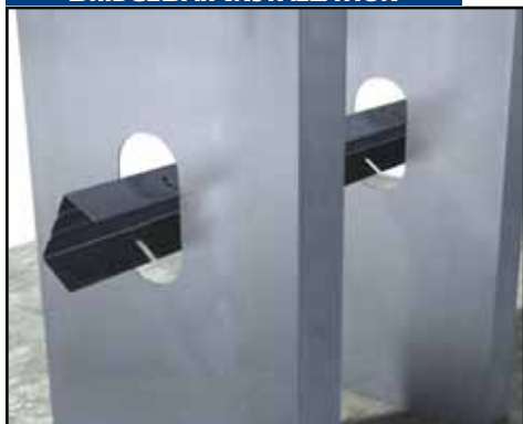
Run BridgeBar through stud punchouts.
