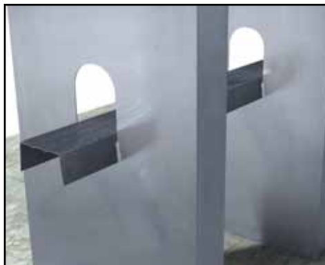
Locate grooves at bottom of punchout and press down into place.
