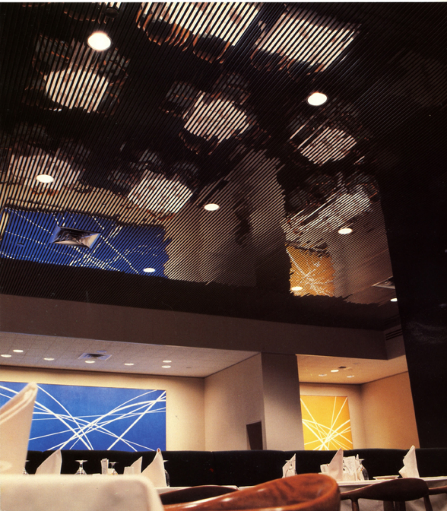
A mirror-finished slat ceiling shaped and assembled by Milgo for an employee dining facility in the Mobil Building, New York City, New York
