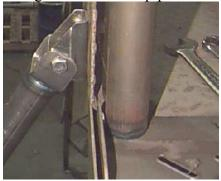
3. Using the angle indicator set the brace to the required angle\*, when setting this angle keep the brace plane 90 degrees to the platform kickplate (small adjustment may be made using the lower bracket assembly). \* When using angle indicator, subtract required angle from 90 degrees, this will give the angle from horizontal.
