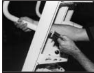
Bolting Handrails to Stair
