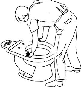
Unplug floor waste opening. Gently place the bowl, right side up, in position with the toilet mounting bolts protruding through the holes in the china base. Press down, with a slight twisting motion, on the top center, with your full weight. Make sure the bowl is as level as possible. If needed, you can use wedges under the bowl to help leveling. Put the washers (Marked: This Side Up) and nuts on the bolts. Tighten them evenly and snugly.
