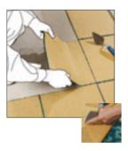
Whether laying mosaic floor or fixing to walls, the steps of the procedure for Opus Romano are the same as described previously for the application of paper-faced mosaic. We recommend **slicing** the paper **into strips 2 - 3 tesserae wide** in the same direction as the lines on the paper, before wetting the paper.
