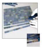
Before laying finishing tesserae, if required, it is advisable to prepare the necessary number of mosaic strips, cutting the sheet with a cutter in a vertical direction following the thicker mesh strand. Once the various strips have been cut, trim off the mesh threads that protrude laterally and then arrange the tesserae of each strip, cutting a minimum amount of mesh between one tessera and the next to facilitate the creation of curves on a flat plane.
