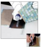
In the case of paper-mounted mosaic, prepare the material by cutting the sheet into strips of tesserae following the grain, using a smooth trowel. The support must be cut with care, leaving only a small area of paper on the tesserae in such a way that they maintain a certain degree of mobility and can adapt to follow rounded surfaces while they are being laid.
