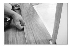
Position the panel onto the already installed row; slide the panel under the obstruction. It's a good practice to pre-fit the panel to make certain it will slide back into place before applying adhesive.
