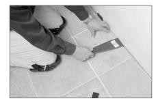
Saw each panel in the last row accordingly and fit them into place using the pull bar. Then add the spacing wedges to hold the joints firmly in place and to create the required expansion gap between these last panels and the wall.
