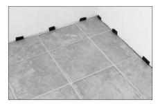
As with all tile formats, the best appearance is achieved by "balancing" the tiles at both the end and side walls. This can be accomplished by finding the centerline of the work area and adjusting the panels to provide equal size tiles at all walls.
