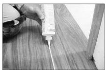
Separate the panels to completely expose the groove. Apply a light coat of Mannington MegaGlue<sup>™</sup> onto the groove; slide the last row panel back into position. If necessary, use a last board puller to position the panel and lightly tap panel to close any gap. Wipe off any excess glue.
