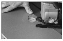
First measure the diameter of the obstacle. Then measure that distance from the edge of the plank to be installed around the obstacle so you know where to drill the hole. Drill holes in the floor plank 5/8" larger in diameter than the obstacle and the correct distance from the edge of the plank. If the hole is near the edge of the plank, cut the plank at a 45° angle to both sides of the hole.
