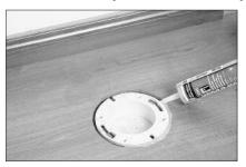
When installing laminate planks in a bathroom, remove the toilet and fit flooring to within 5/16" of the toilet flange. Fill this expansion gap with high-quality silicone caulk.
