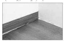
Install T-Moldings and Wall Base over the silicone caulk-filled expansion gaps. Nail Wall Base directly into the wall, not into the laminate flooring. Fill the expansion gap between planks and tub with a high-quality silicone caulk then install the profile into the wet silicone. In areas where a square edge profile cannot be installed, completely fill the 5/16" expansion gap with silicone caulk.
