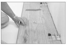
Slightly angle the side tongue profile of this panel into the side groove of the panels in the first row, and with a slight wiggling action, press tongue into groove and lower into position. (The tape will secure the previously assembled panels together.) If necessary, tap with the heel of your hand to close any minor gaps.
