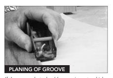
If there are obstacles (door casings, toe kicks, radiators) that prevent the last row panels from being angled into position, it is necessary to lightly plane or sand off a bit of the locking profile of the groove and tongue.
