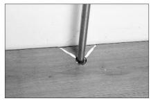
Now you will have two separate plank pieces to enable positioning around the obstacle. Apply a liberal amount of MegaGlue™ adhesive to the cut pieces and press into place. Tighten with a pull bar and wipe away excess adhesive with a clean, damp cloth.
