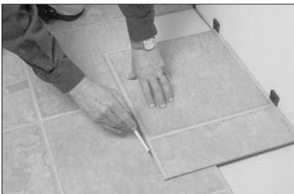
The last row of tile panels should be the same width as the first row. To scribe the last row of panels into place accurately, align the panel over the last installed row of panels and scribe to fit. Be certain to provide the required expansion gap.
