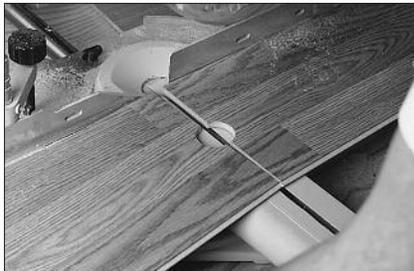
If the hole is near the center of the plank, cut perpendicular to the long edge, going directly through the middle of the hole.
