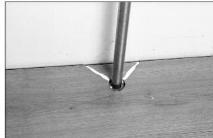
Now you will have two separate plank pieces to enable positioning around the obstacle. Apply a liberal amount of MegaGlue™ adhesive to the cut pieces and press into place. Tighten with a pull bar and wipe away excess adhesive with a clean, damp cloth.
