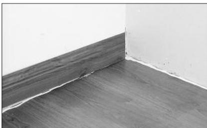
Install T-Moldings and Wall Base over the silicone caulk-filled expansion gaps. Nail Wall Base directly into the wall, not into the laminate flooring. Fill the expansion gap between planks and tub with a high-quality silicone caulk then install the profile into the wet silicone. In areas where a square edge profile cannot be installed, completely fill the  $\frac{5}{16}$ " expansion gap with silicone caulk.
