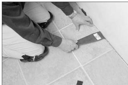
Saw each panel in the last row accordingly and fit them into place using the pull bar. Then add the spacing wedges to hold the joints firmly in place and to create the required expansion gap between these last panels and the wall.
