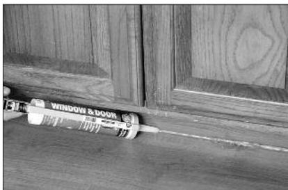
To finish installations in a high-humidity or wet environment, the expansion gaps at all vertical surfaces such as walls, cabinets, etc., must be filled with high-quality silicone caulk.
