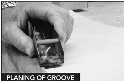
If there are obstacles (door casings, toe kicks, radiators) that prevent the last row panels from being angled into position, it is necessary to lightly plane or sand off a bit of the locking profile of the groove and tongue.
