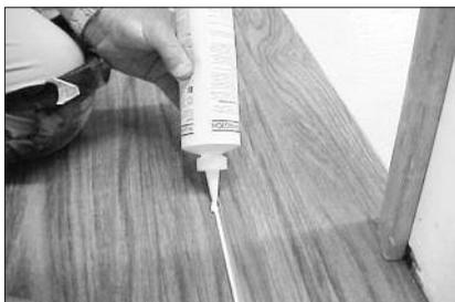
Separate the panels to completely expose the groove. Apply a light coat of Mannington MegaGlue™ onto the groove; slide the last row panel back into position. If necessary, use a last board puller to position the panel and lightly tap panel to close any gap. Wipe off any excess glue.
