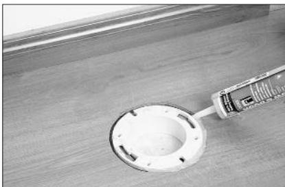
When installing laminate planks in a bathroom, remove the toilet and fit flooring to within  $\frac{5}{16}$ " of the toilet flange. Fill this expansion gap with high-quality silicone caulk.
