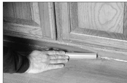
Install Quarter Round moldings directly into the wet silicone caulk.
