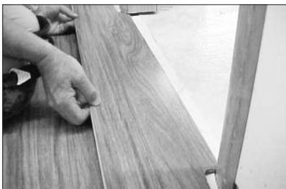
Position the panel onto the already installed row; slide the panel under the obstruction. It's a good practice to pre-fit the panel to make certain it will slide back into place before applying adhesive.
