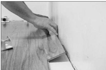
The last row of panels will more than likely need to be cut to fit. If not, it is still necessary to cut off the groove profile to provide a full plank thickness at the wall. If nothing prevents angling this last row of planks into position, proceed as normal to complete the installation.
