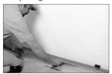
Before starting to glue planks, dry-lay the entire first two rows on top of the selected underlayment. Begin in the upper right corner of the work area with the groove side of the planks facing the wall. Place spacing wedges along the walls on both the ends and sides of all planks.
