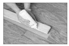
Always use Mannington adhesive and sundry products. When employing the floating method, apply adhesive to the bottom of the groove on the repair plank. For the glue-down method, spread the appropriate amount of UltraSpread Mastic<sup>TM</sup> with the correct V-notched trowel.
