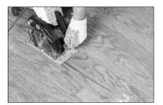
To remove the plank you must cut it with a circular saw. Set saw to precise depth of plank. Cut diagonally from one corner hole to the opposite corner hole to create an "X" in the damaged plank. Follow directions below to remove cut planks.
