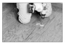
To replace an entire damaged plank, begin by drilling four 1/2" holes in the damaged plank approximately 1/4" away from all four plank corners. Use extreme caution when drilling to prevent damage to adjoining planks. It's a good idea to mark your cutting path before drilling or sawing into the damaged plank.
