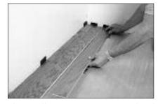
The installation sequence is critical and provides stability to the first two rows. Closely follow the next several instructions to obtain the proper gluing sequence for the first few rows of planks. To start, glue the first plank in the second row to the first plank in the starter row, and so on.
