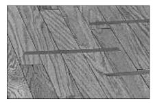
After several rows of planks are down, secure the rows using non-marring, releasable blue painters tape. Do not allow the tape to remain on the planks longer than required. Repeat this process as the installation progresses.
