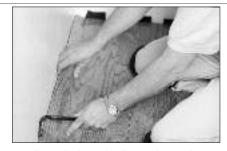
Install cut planks and pull into place with a pry bar. Install spacing wedges between planks and wall. Allow floor to dry for a minimum of 12 hours before removing all spacing wedges and allowing foot traffic. Sweep the floor to remove all dust and dirt, taking care not to scratch the finish.
