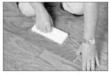
Slide the repair plank into place using a tapping block, first inserting the side with 3" cut off the tongue. Wipe away any excess glue with a clean dampened cloth or with a Mannington glue scraper. Weight the repair plank and avoid active foot traffic for approximately 12 hours after the repair has been completed.
