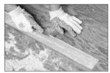
Once the plank is thoroughly removed, clean the tongue-and-groove joints of the surrounding planks with a sharp chisel.
