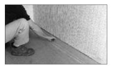
Snap a chalk line from these points, parallel to that wall and perpendicular to the adjacent walls. Since most walls are not straight, the edge of some planks may have to be trimmed along the wall or cut to fit.
