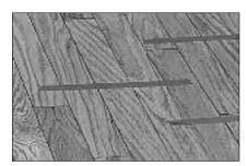
After several runs of planks are down, use strips of non-marring, releasable blue painters tape to hold the planks securely. Repeat this process as the installation progresses.
