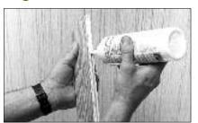
In a floating floor installation, the flooring is NOT nailed or glued to the underlayment, but is glued in the plank's groove only. Apply Mannington MegaGlue adhesive to the bottom of groove along the entire length and on the end of each plank. **Do not completely** fill the groove with adhesive.
