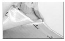
Install one sheet of AquaBarrier™ II underlayment net along the starting wall. Unroll only one sheet at a time during plank installation to prevent damaging the underlayment. If any part of the AquaBarrier II underlayment is punctured or damaged during installation, seal the area with duct tape.
