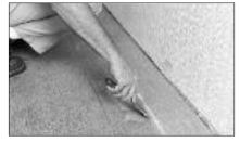
Spread Mannington UltraSpread Mastic from the chalk line out to the width of two planks with a minimum 3/16" x 5/32" V-notched trowel. You can start laying planks immediately into wet adhesive; however, for optimum performance Mannington recommends allowing the adhesive to set for 30 minutes.
