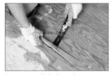
To remove cut planks, loosen by prying up at saw cut with a chisel or small pry bar.
