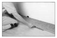
Glue the next plank to the plank in the previous row. Apply adhesive only to the width end of the plank. Tap the planks together carefully with a tapping block and hammer. Remember to continually remove adhesive squeezed up between the joints with a glue scraper or a clean damp cloth.
