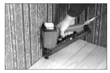
Face nail or tack each final plank into place with the pneumatic stapler. Install the molding and retain a few leftover planks in case a repair is ever required. Do not use manual nailers on any Mannington Hardwood Floors maple flooring or on any Tradewinds Collection or Caspian LOCKnGO. Bamboo flooring should not be stapled. Sweep floor to remove all dust and dirt. Take care not to scratch the finish.
