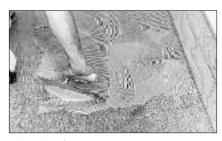
When the first two starter rows are secure, spread 2-1/2' to 3' of adhesive across the length of the room. (Never spread more adhesive than can be covered in approximately three hours). If the adhesive has set and will not transfer to the back of the plank, scrape up the adhesive and apply fresh UltraSpread Mastic™ adhesive.
