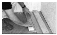
The precise engineering of our UltraFit™ tongue-and-groove system creates a very stable floor. But you MUST make a good connection. Use a tapping block to tap the planks together until the tongue and groove "snap" into place.
