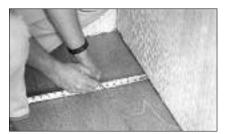
Select a starter wall. An outside wall is best because it's more likely to be straight and square with the room. Measure out from this wall, at each end, the width of two planks.
