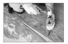
Use a chisel and a hammer to remove any remaining damaged plank pieces.
