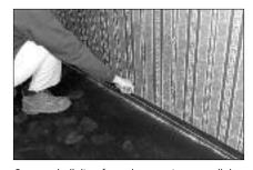
Snap a chalk line from these points, parallel to the wall and perpendicular to the adjacent walls. Since most walls are not straight, the edge of some planks may have to be trimmed along the wall or cut to fit. It is not necessary to leave an expansion space for Mannington 9/16," 1/2," and 3/8" thick planks. **Bamboo** requires a 5/16" expansion space for a nail down installation.
