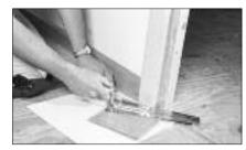
Undercut all doorcasings 1/16" higher than the thickness of the flooring and underlayment to be installed. Place a scrap piece of plank and a sheet of underlayment against the doorcasing to act as a guide, and cut the doorcasing with a hand saw or power jamb saw set to the correct height.
