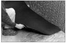
For the staple-down and nail-down methods, cover the subfloor with red rosin paper or any other suitable lining material. This will help keep dust away from the wood floor, retard moisture from below, and may help prevent squeaks from occurring. There is no complete moisture barrier system, however, for naildown and staple-down applications. Maximum wood subfloor moisture should never exceed 14%.
