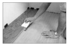
Use a tapping block and a hammer to push glued planks together until no gaps are seen. Immediately wipe away any excess adhesive with a clean damp cloth.
