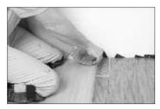
At the end wall use a pry bar, if needed, to pull the ends of the planks tight. Continue laying the floor on top of the selected underlayment, working right to left, laying plank after plank, row after row, tapping the planks together as you go. Be sure to continue using 5/16" spacing wedges at all walls and obstructions throughout the installation.
