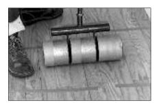
Thoroughly roll the flooring in both directions using a clean, three-section 100-lb floor roller. Clean with any urethane adhesive cleaner.
