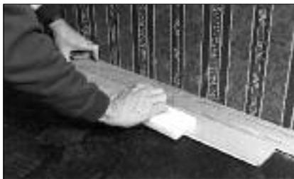
*The precise engineering of our UltraFit™ tongue-and-groove system delivers a very stable floor. But you MUST make a good connection. Use a tapping block to tap the planks until the tongue and groove “snap” into place.*
