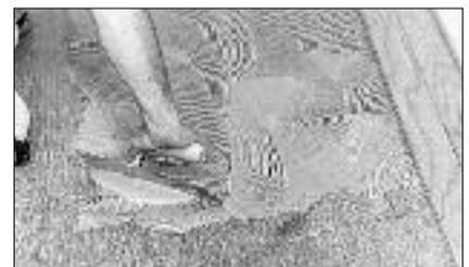
When the first two starter rows are secure, spread 2-1/2' to 3' of adhesive across the length of the room. (Never spread more adhesive than can be covered in approximately three hours). If the adhesive has set and will not transfer to the back of the plank, scrape up the adhesive and apply fresh UltraSpread Mastic™ adhesive.
