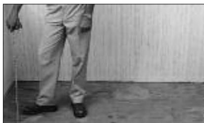
After deciding the direction in which the planks will run, measure the width of the room (the dimension perpendicular to the direction of the flooring). The last row of flooring should be no less than 1-1/2" wide. If it is less, we recommend cutting the starter row narrower. This will require extra cutting but it will make the rest of the installation easier and faster.
