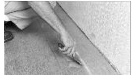
Spread Mannington UltraSpread Mastic from the chalk line out to the width of two planks with a minimum 3/16" x 5/32" V-notched trowel. You can start laying planks immediately into wet adhesive; however, for optimum performance Mannington recommends allowing the adhesive to set for 30 minutes.
