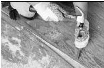
Use a chisel and a hammer to remove any remaining damaged plank pieces.
