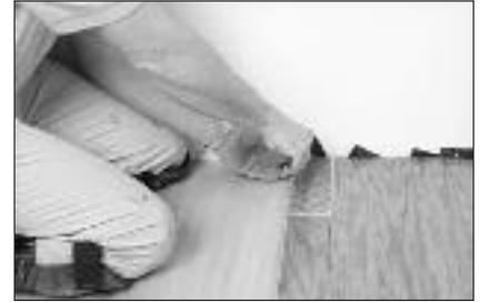
At the end wall use a pry bar, if needed, to pull the ends of the planks tight. Continue laying the floor on top of the selected underlayment, working right to left, laying plank after plank, row after row, tapping the planks together as you go. Be sure to continue using 5/16" spacing wedges at all walls and obstructions throughout the installation.
