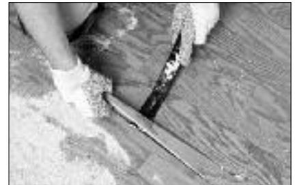
To remove cut planks, loosen by prying up at saw cut with a chisel or small pry bar.
