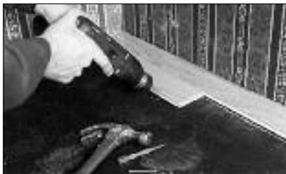
*After the first row is complete, adjacent rows should also be predrilled in the nail pocket and secured with finishing nails set at 45°. Rows of flooring will need to be installed in this manner until flooring planks are a sufficient distance away from the wall to accommodate the stapler. Stapling schedule is every 6" to 8" on center.*
