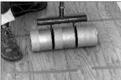
Thoroughly roll the flooring in both directions using a clean, three-section 100-lb floor roller. Clean with any urethane adhesive cleaner.
