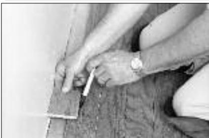
The last row will most likely require cutting to width but it should be no less than 1-1/2" wide. To do this, lay the plank on top of, and edge-to-edge with, the plank in the next-to-the-last row. Trace the wall contour on the last plank using a scrap piece of plank and cut as required.
