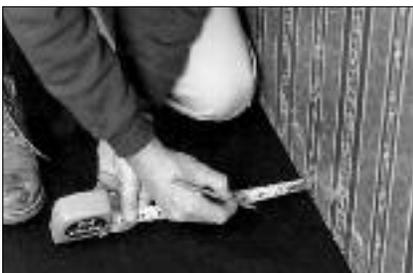
Select a starter wall. An outside wall is best because it's most likely to be straight and square with the room. Measure out from this wall, at each end, the width of the plank plus 1/4."
