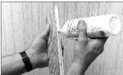
In a floating floor installation, the flooring is NOT nailed or glued to the underlayment, but is glued in the plank's groove only. Apply Mannington MegaGlue adhesive to the bottom of groove along the entire length and on the end of each plank. **Do not completely fill the groove with adhesive.**
