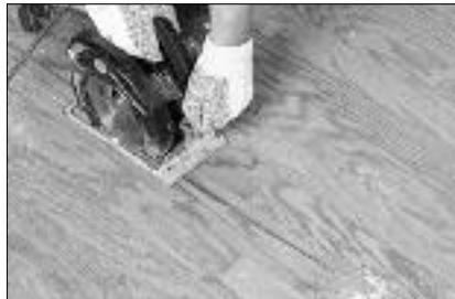
To remove the plank you must cut it with a circular saw. Set saw to precise depth of plank. Cut diagonally from one corner hole to the opposite corner hole to create an "X" in the damaged plank. Follow directions below to remove cut planks.
