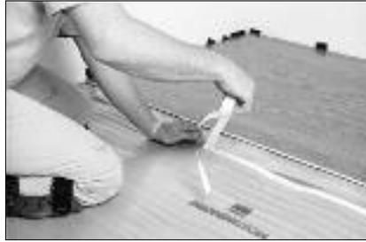
Glue the next plank in the same row to the previously glued plank from the previous row. Apply adhesive to both the length and width edges of the plank.
