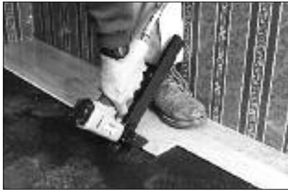
Using the Mannington Spotnails Floor Monster stapler, with the proper adapter attached (see stapler instructions for proper setup), continue to staple new planks every 6" to 8" on center, fastening the ends of the planks approximately 2" from each end.
