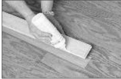
Always use Mannington adhesive and sundry products. When employing the floating method, apply adhesive to the bottom of the groove on the repair plank. For the glue-down method, spread the appropriate amount of UltraSpread Mastic™ with the correct V-notched trowel.
