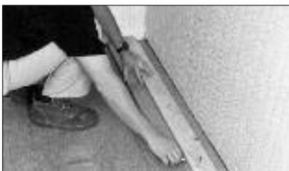
Install the first row of starter planks and secure into position with the tongue facing the starter wall. Proper alignment is critical, misaligned starter rows can ruin the entire installation. It may be helpful to firmly secure a straight edge along the chalk line as a guide; this also helps to prevent planks from shifting in the wet adhesive. Or else, top nail the first row with finishing nails (wood subfloor) or sprig/pin nails (concrete subfloor).
