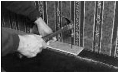
*Install the first row of planks by laying the tongue edges on the chalk line. Proper alignment is critical. Misaligned starter rows can ruin the entire installation. Secure each plank to the subfloor using a pneumatic brad tacker or with finishing nails. Drill pilot holes through the face of each plank (in dark grain) if using finishing nails.*
