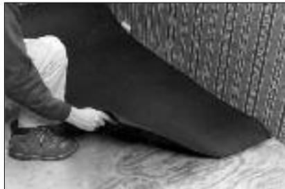
For the staple-down and nail-down methods, cover the subfloor with red rosin paper or any other suitable lining material. This will help keep dust away from the wood floor, retard moisture from below, and may help prevent squeaks from occurring. There is no complete moisture barrier system, however, for nail-down and staple-down applications. Maximum wood subfloor moisture should never exceed 14%.
