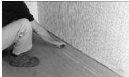
Snap a chalk line from these points, parallel to that wall and perpendicular to the adjacent walls. Since most walls are not straight, the edge of some planks may have to be trimmed along the wall or cut to fit.
