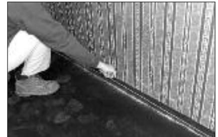
Snap a chalk line from these points, parallel to the wall and perpendicular to the adjacent walls. Since most walls are not straight, the edge of some planks may have to be trimmed along the wall or cut to fit. It is not necessary to leave an expansion space for Mannington 9/16", 1/2", and 3/8" thick planks. **Bamboo requires a 5/16" expansion space for a nail down installation.**
