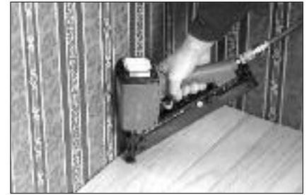
Face nail or tack each final plank into place with the pneumatic stapler. Install the molding and retain a few leftover planks in case a repair is ever required. **Do not use manual nailers on any Mannington Hardwood Floors maple flooring or on any Tradewinds Collection or Caspian LOCKnGO. Bamboo flooring should not be stapled.** Sweep floor to remove all dust and dirt. Take care not to scratch the finish.
