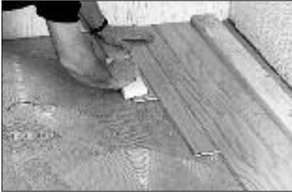
Place planks into position on top of adhesive and tap into place with a tapping block. Avoid clustering the end joints. Stagger random lengths so that end joints are no closer than 6."
