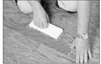
Slide the repair plank into place using a tapping block, first inserting the side with 3" cut off the tongue. Wipe away any excess glue with a clean dampened cloth or with a Mannington glue scraper. Weight the repair plank and avoid active foot traffic for approximately 12 hours after the repair has been completed.
