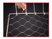
2.2 Thread ends of installation rope through permanent crimp and press with pliers. Trim excess installation rope.
