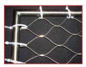
1.3 Trim excess diamonds from opposite end of mesh panel using wire cutter and install self-locking end ferrules.
