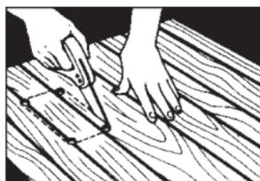
Transfer these measurements to panels for cutting. If using a handsaw or table saw, mark and cut the panels face up. If using a portable circular saw or sabre saw, mark and cut panels face down. Cut-outs for door and window sections, electrical switches and outlets or heat registers require careful measurements.
