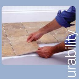
Plywood is the preferred structural panel sub-floor under backer board when applying ceramic tile, according to the Tile Council of America and National Tile Contractors Association.
