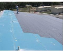
Sark is a firm believer in self-adhered roof systems. "It dries in a building quickly. It's simple to install. And the dry-in is secure. You don't have to worry about wind blowing the felts up. And with the self-healing characteristics of the membrane, mechanical penetrations won't leak."
