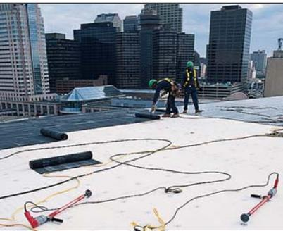
reduces the chances of board fracture that often occurs at the base of fastener stress plates. This is especially true with a fully adhered torch down application such as this.” Additionally, the combination of embedded glass matt surfacing and a water resistant treated core make DensDeck® Roof Board very conducive to adhesion.
