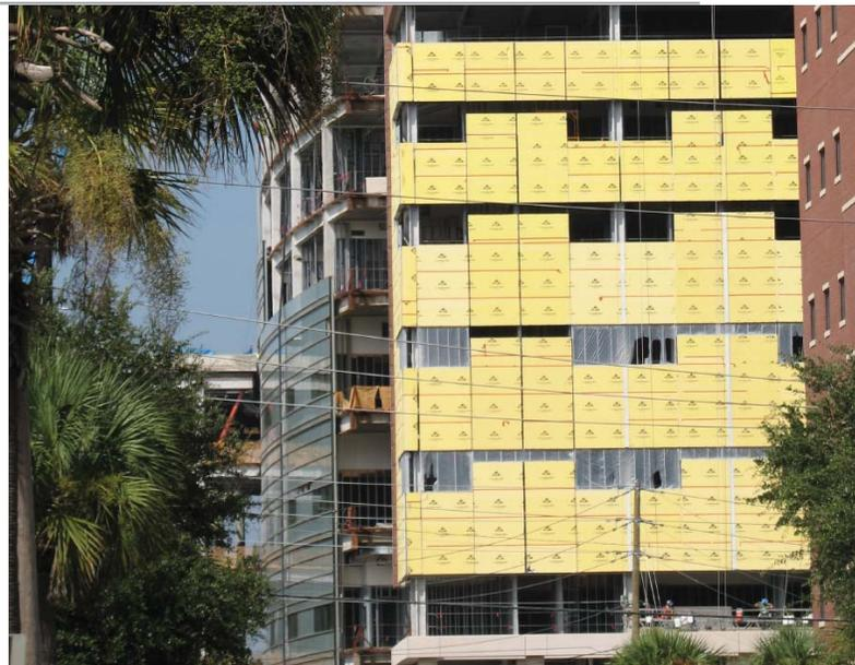
hanging DensArmor Plus panels about *four months before* we would have hung traditional paper-faced gypsum board. Cascading rain had no effect. After eight months exposure to the elements, the fiberglass mat panels looked like the day we put them up. And, the no-paper design leaves no food for mold.”
