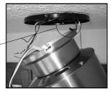
With fan safely suspended by hook, make wire connections with wire nuts included in fan hardware package as described in the control installation instructions. If using the optional #003 or #004 control, the receiving unit should be connected at this time and placed inside the hugger canopy.
