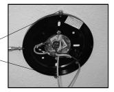
**(6)** Lift fan body and hang from ceiling plate hook. The hook should go through one of the closed holes in the hugger canopy.
